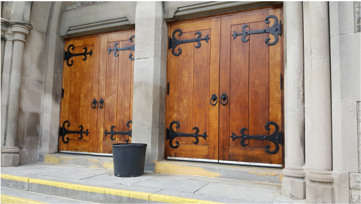
Refinished sanctuary main doors.
